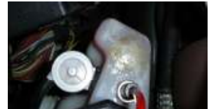
Bulkhead Fitting Installed in Washer Tank.
