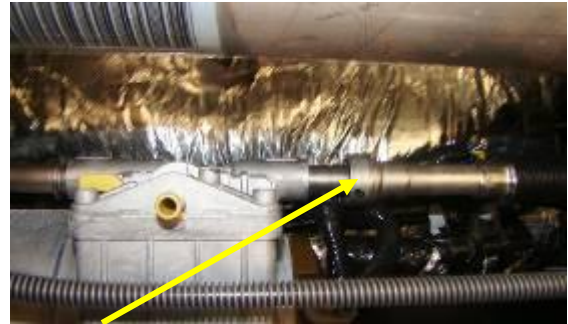
Figure 15 View From Below
