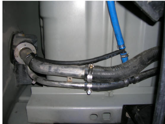
(Fig. 8) Photo shows final installation of fill hose and vent line hoses on vehicle's fill spout. Note the 1/4" Vent Kit Assembly hose is securely fastened to the fill spout. The 1/4" vent is necessary to prevent vacuum build-up in your TITAN™ fuel tank.
