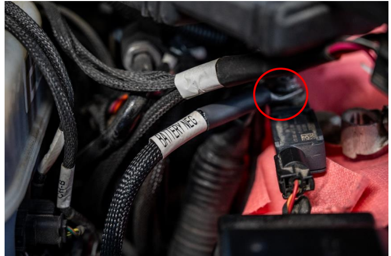
Figure 40: Heater ground cable installed onto battery (-) negative terminal.
