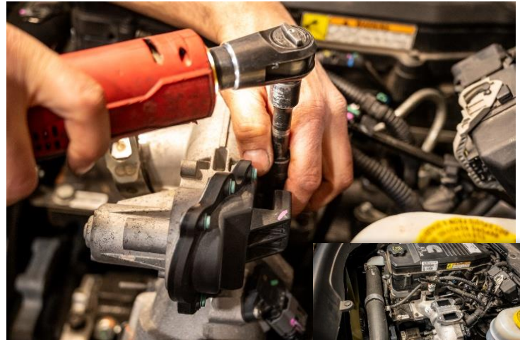
Figure 12: Removal of the four 10MM bolts retaining the EGR Valve. Discard stock gaskets.
