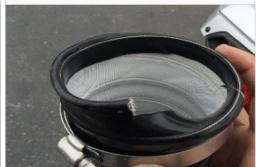
25. Insert one end of the Duct (N) and Hose Clamp (O) onto the Air Tube (M). Tighten the hose clamp at the air tube. Bring the other end towards the opening on the Particle Separator (A). Note the length on the duct you want to cut. We recommend cutting the duct an extra 3" longer so that the ends, along with any wire and strings, can be folded in for a cleaner look.
