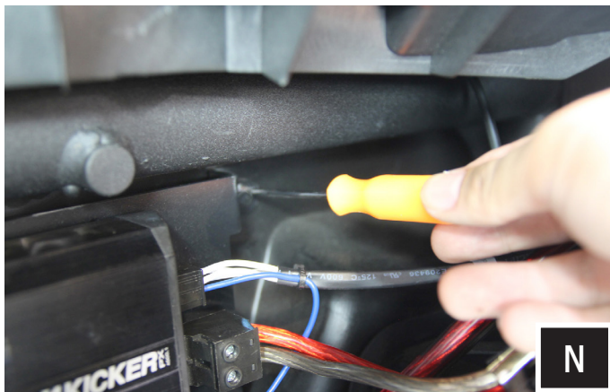
N. Make a pilot hole with a pick tool through the top right screw hole in the amp plate and push all the way through the vehicle panel.
