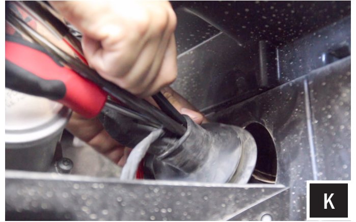
K. Unwrap the tape from rubber grommet and feed the power/ground wire for the Amp through the grommet as well as the rear speaker harness H1151.
