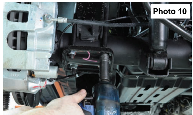
Remove the factory u bolts and hardware.
